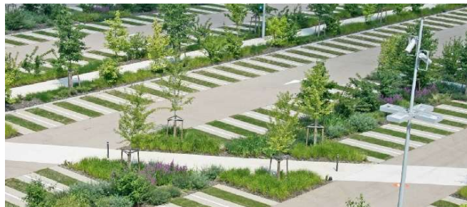
IMAGE 24 – Example of permeable car parking with rain garden solution, footpaths and trees
